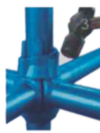
(3) Tightening with a hammer
